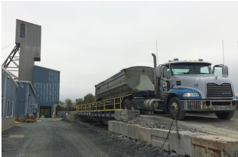
Truck scale and shaft headframe
